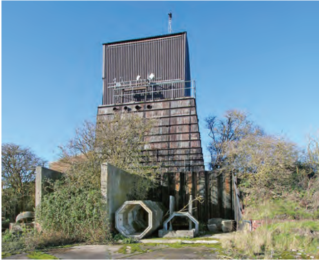
P2 – the corrugated metal sheeting was added partially to hide Chevaline Polaris. The octagonal concrete segments in front of the stand are part of the 1/6 size Blue Streak silo
